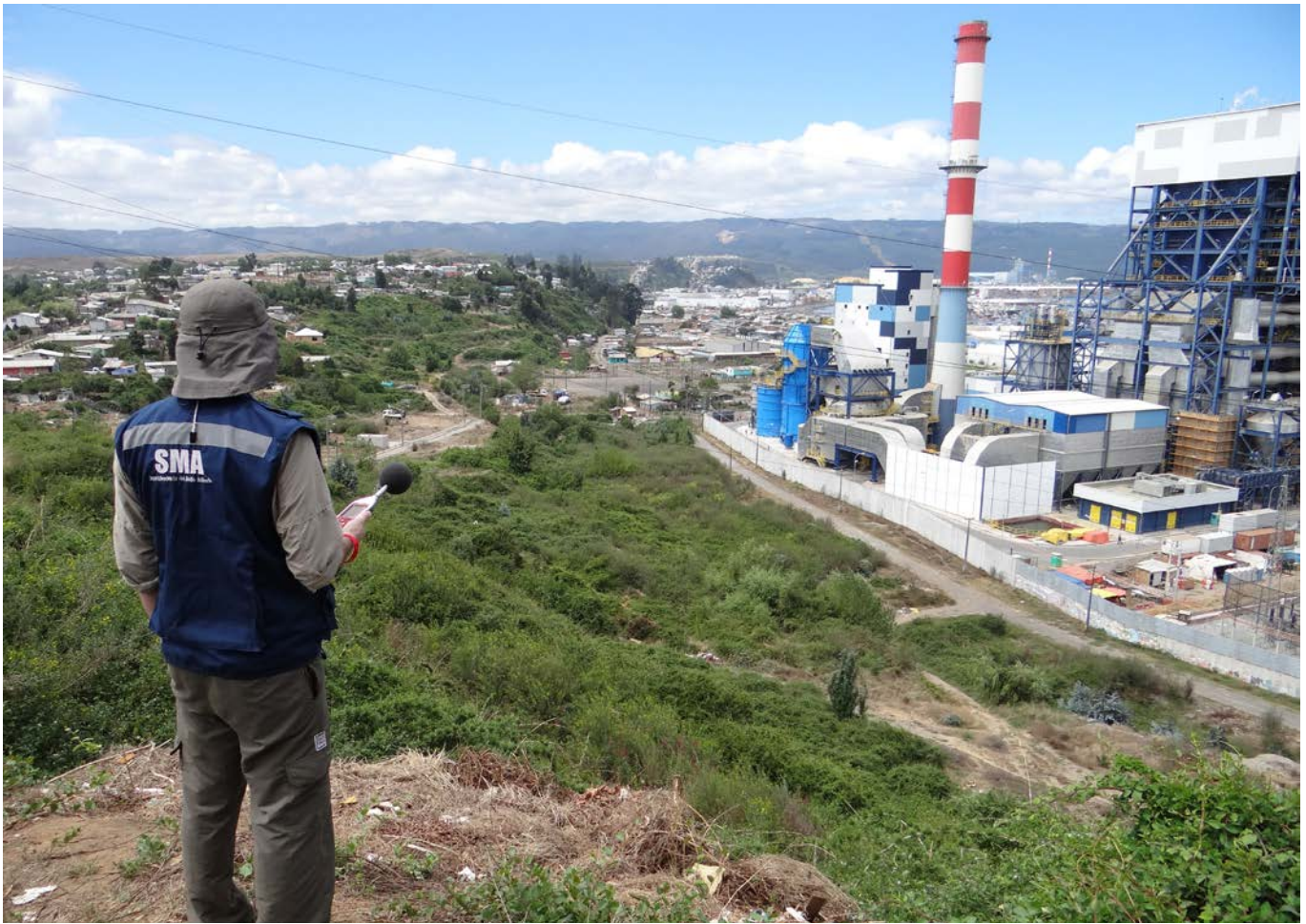
Bocamina Thermo Power Generation Plant
